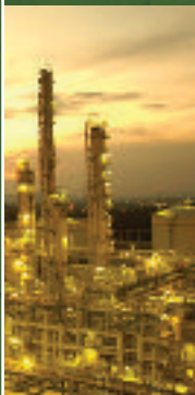
Petrochemicals and Refinery
